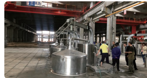
Xiaojiailou's new pits in operation
