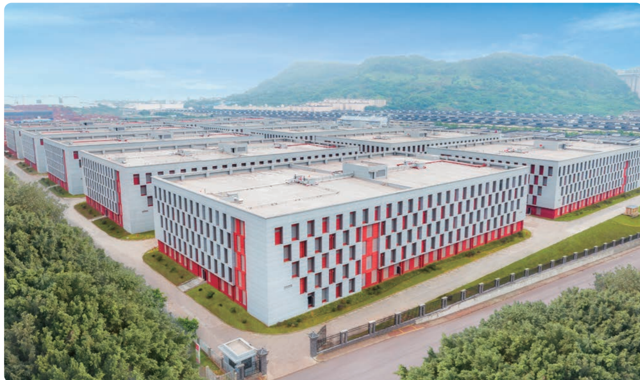
300,000-Ton Pottery Jar Aging Spirit Room Project (Phase I)
