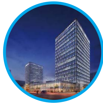
上海张江高科技园区中区C-7-2
